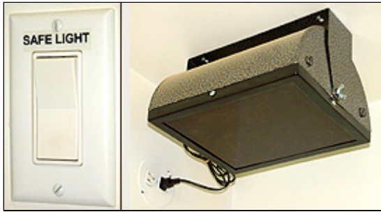
Don't locate your safe light switch close to the room's main white light switch to avoid accidentally turning on the wrong light.
