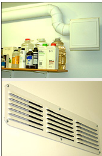
A light-tight fresh air inlet on the dry side and an extractor fan located above the wet side ensure a continuous supply of fresh air.
